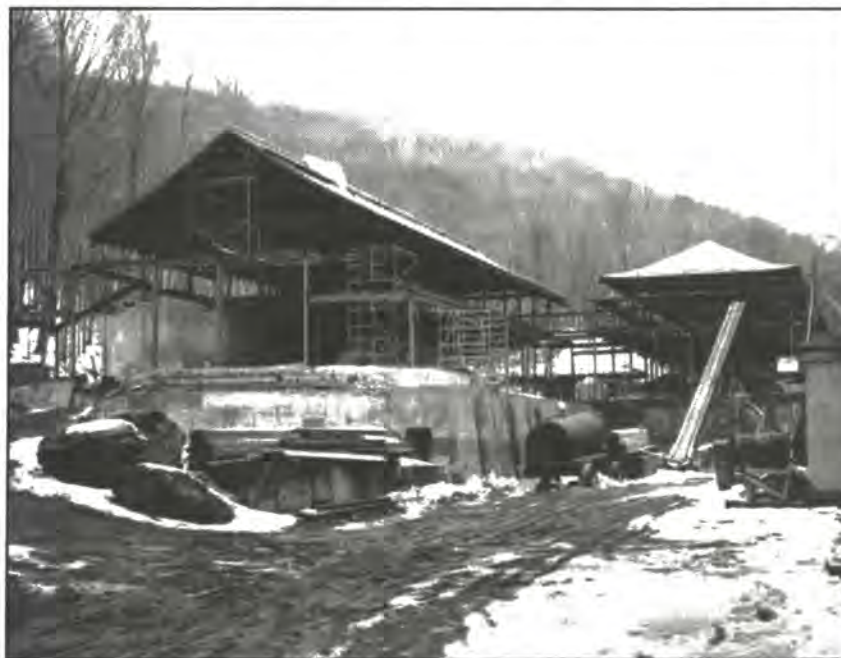
The monastery under construction.
